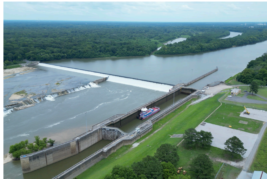
Demopolis Lock and Dam. Source: Port of Mobile
